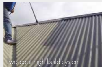
Two coat high build system
